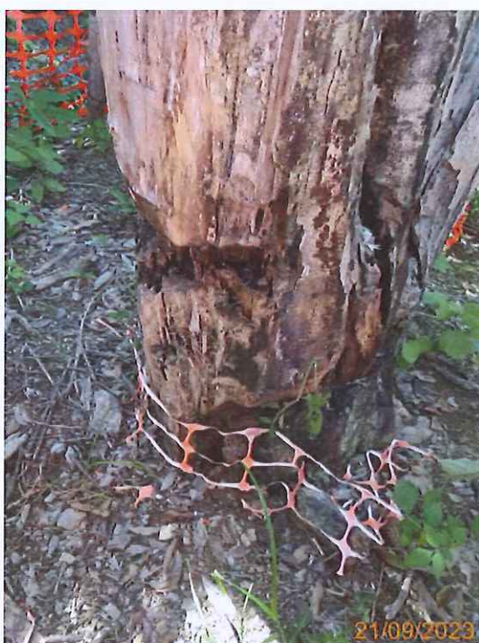
8: U041_Wood damaged by termite
